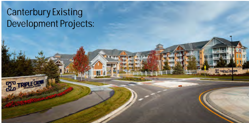
Phase I Completed/Phase II Under Construction
